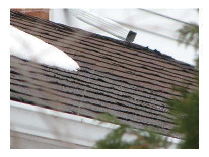
Valley flashing is showing evidence of accelerated deterioration. Asphalt roof valley will deteriorate faster than the remaining roof surface due to continuous wear from rain water redirected to this area. Metal valleys should be considered during the next roof resurfacing project. Water penetration is possible at this area. Strongly recommend immediate action. Repair or replace as required.
