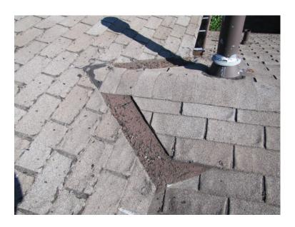
Missing shingles water penetration is possible at this area. Continuation of this condition could lead to water damage. Continuation of this condition could lead to structural damage. Strongly recommend immediate action. Consult a specialist for further evaluation and recommended action. Recommend repair.
